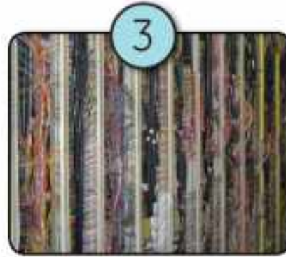
Thousands of individual copper wires from switchyard
