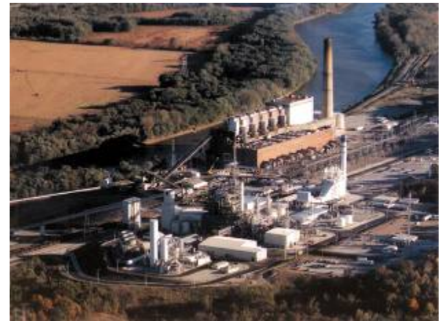
PSI Energy Wabash River IGCC Power Plant
